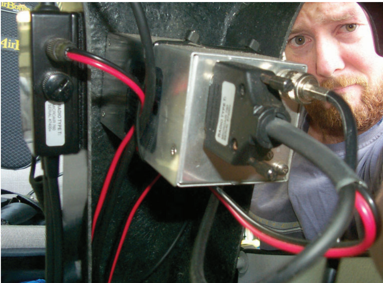
PHOTO SHOWS WIRE ROUTING AFTER INSTALL.
